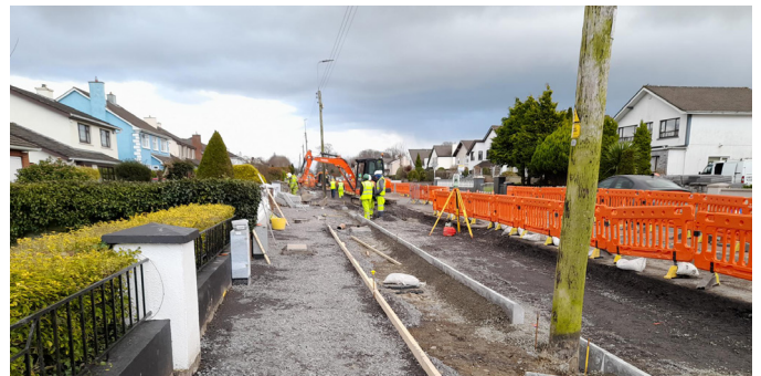
N63 Majors Well Road footpath installation
